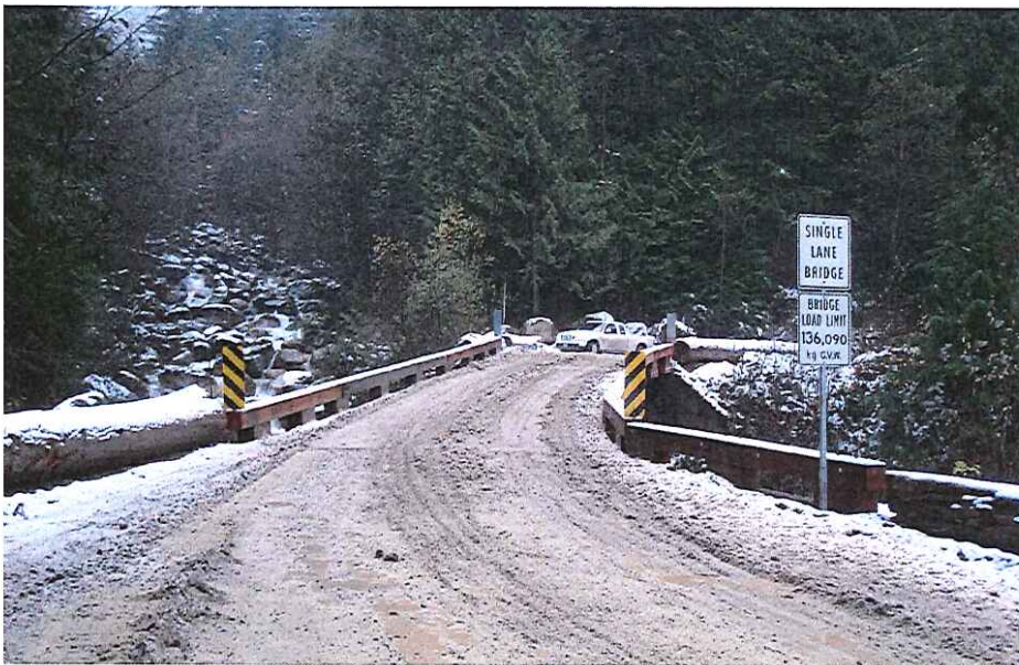
CK-2021 Approach Right Bank
