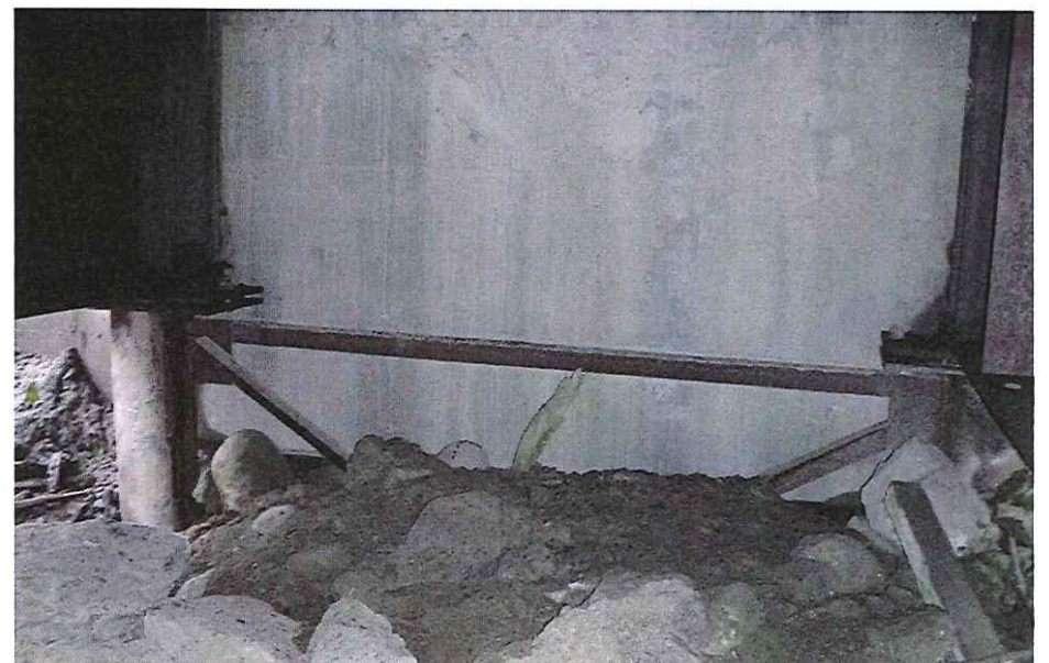
CK-2021 Abutment Right Bank
