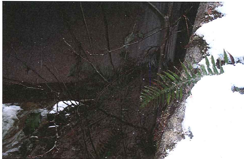
CK-2021 Side View of Abutment Right Bank
