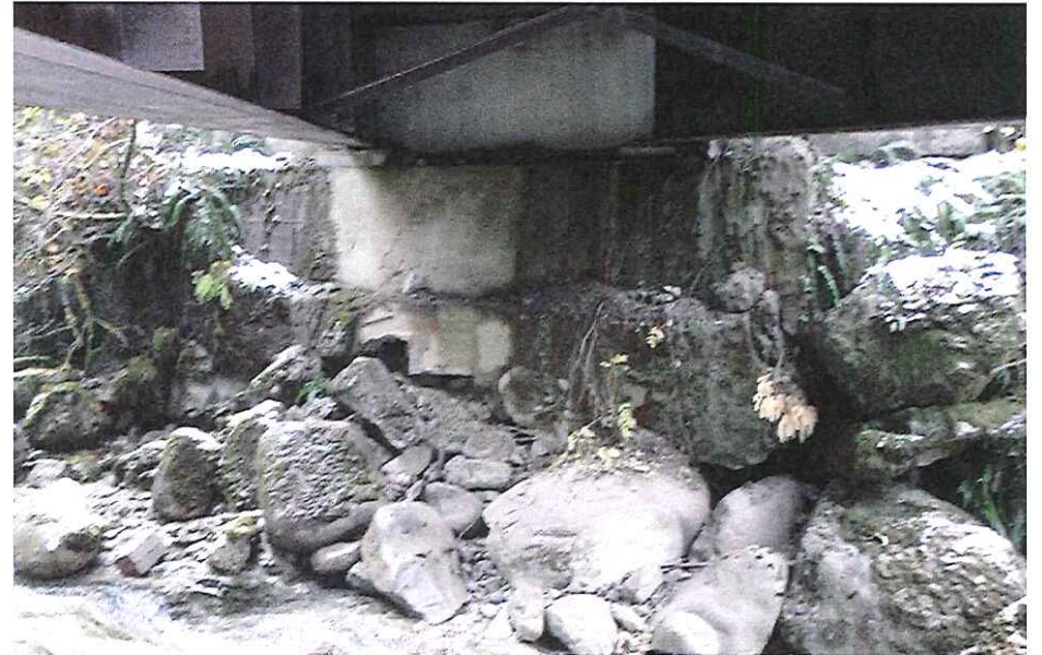
CK-2021 Abutment Left Bank
