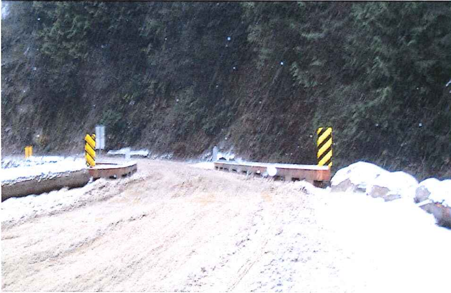
CK-2021 Approach Left Bank
